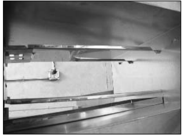
14. Install the upper air panel assembly.
